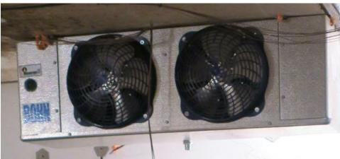
Figure 173 – Walk-in Unit Cooler
