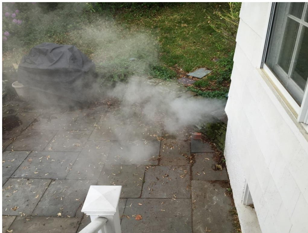
Figure 25: Condensate from a Condensing Boiler
